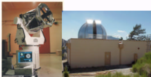
1-m OCTL Facility (under construction)
